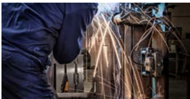
Welding of frame
