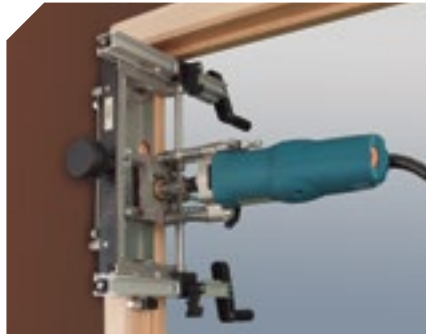
Making the upper recess on the frame.
