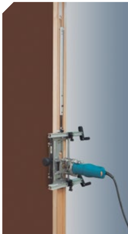
Making the second recess on the frame.
